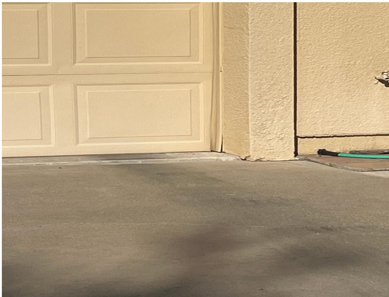
Embers can access garage space through separating jamb
